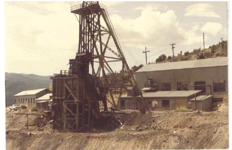
Caselton Mine #2 Headframe, Hoist and Compressor Building Circa 1985
