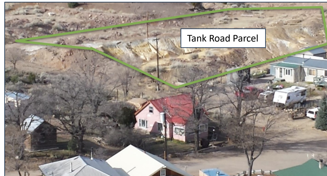
Green boundary shows approximate area of tailings material on the Tank Road Parcel
